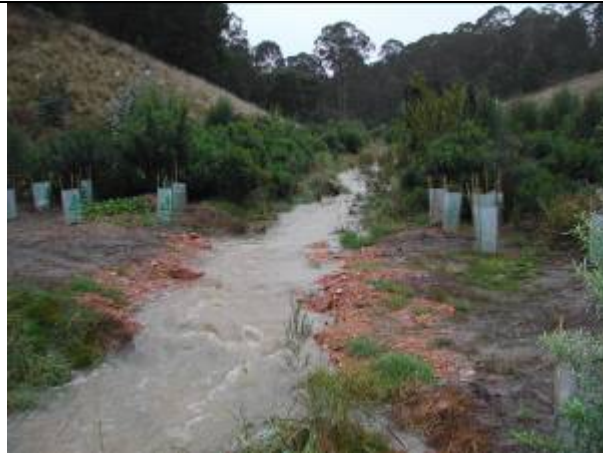
Figure S52. Frenchman's Gully, Lakes Entrance Victoria. This site is the famous Infill Gullies project. Many of its drains, such as this one at Frenchman's Gully, are straight and are designed to get water from the catchment to the lake as quickly as possible and to deprive the alluvial flat of its floodwater. This leaves little time (or space) for water to slow down and drop its sediment (and phosphorus load) (compare the velocity in this figure with that of Figure S53. As urbanisation increases in the catchment, water flow rates and erosion increase and remedial action is needed. Fortunately for this site, the landholders are very aware of this issue and have offered every assistance in getting this restoration project going.
