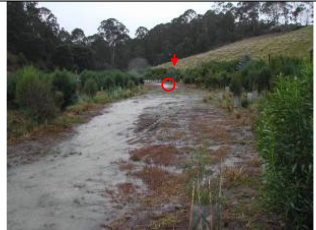
Figure S53. Frenchman's Gully, Lakes Entrance Victoria. The drain (Figure S52) is being progressively blocked and re-directed to meander across the floodplain and re-form its original course as a creek while the gully floor is having its original Warm Temperate Rainforest and Swamp Scrub restored. The water is slowed, spends more time on land and drops more of its sediment load. Immediately downstream (Figures S55, S56), the creek enters a lakeshore swamp before disgorging into the North Arm. The swamp purifies low flows (of nitrogen and dissolved phosphorus), while the rainforest restored to the alluvial flats will treat higher flow events for phosphorus. Over a distance of just 400m (and after only 2 years of growth), these rainforest plantings have stripped 88% of the phosphorus from the groundwater entering the site, before it could go into the North Arm estuary! The red arrow marks the photographic point and the red circle that is shown in Figure S54.
